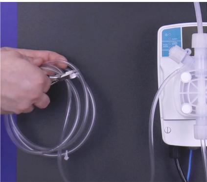
**Step 53:** Using the diagonal pliers, cut the tube so that it is long enough for the chemical bleed off to go into the bucket or stock tank.
