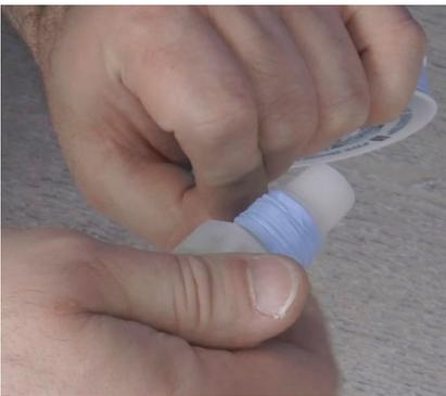
**Step 15:** Take the thread seal tape and wrap it around the threads of the injection valve for the necessary size; either 3/8 or 1/2 inch.
